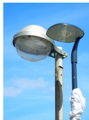
Installation de lampadaire led
